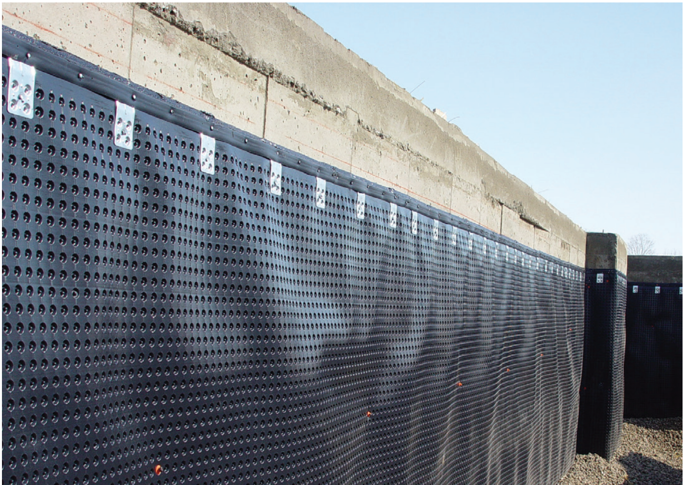
FINISHED INSTALLATION OF PLATON FOUNDATION WRAP
