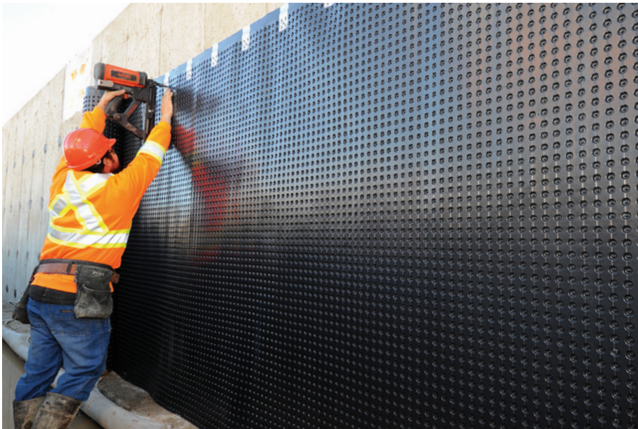
INSTALLING SPEEDCLIPS EVERY 30CM (12")
