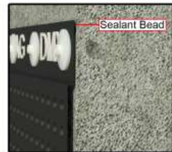
DETAIL 1 Sealant bead to be placed at the top of the flat tab.
